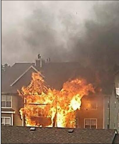
The cause of this fire was due to the prohibited use of a propane bar-b-que grill on an exterior second floor balcony.
